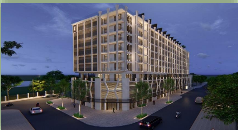
○ TRIBE HOTEL PHNOM PENH PROJECT
